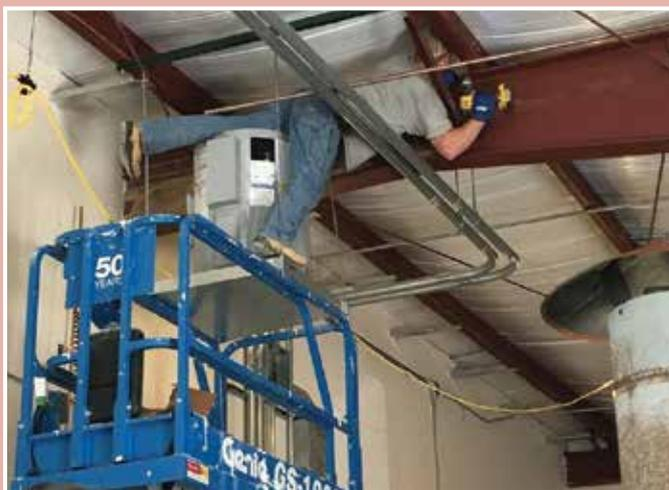
Spotted in the USA a man working on an overhead beam with a power drill. While he has a scissor lift, he has completely left it - a ladder would probably have been a better solution.
