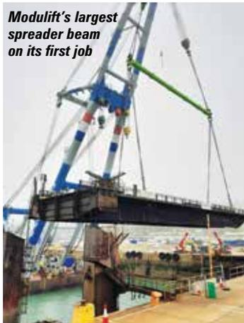
*Modulift's largest spreader beam on its first job*
