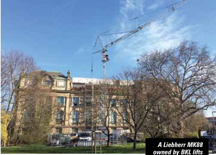
*A Liebherr MK88 owned by BKL lifts components onto the new roof of the Lower Saxony State Museum in Hanover*
