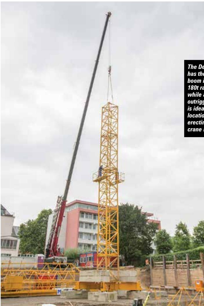
*The Demag AC 160-5 has the longest boom in the 130-180t range, at 68m, while asymmetric outrigger set up is ideal for tight locations such as erecting this tower crane in Bonn*
