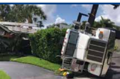
This truck crane overturned in Ft Lauderdale, Florida, earlier this month when two of its outriggers dropped into an underground septic tank. The crane operating company said: "The customer advised that there was NO septic tank, thus making it safe to park in the driveway but there was, in fact, a septic tank."
