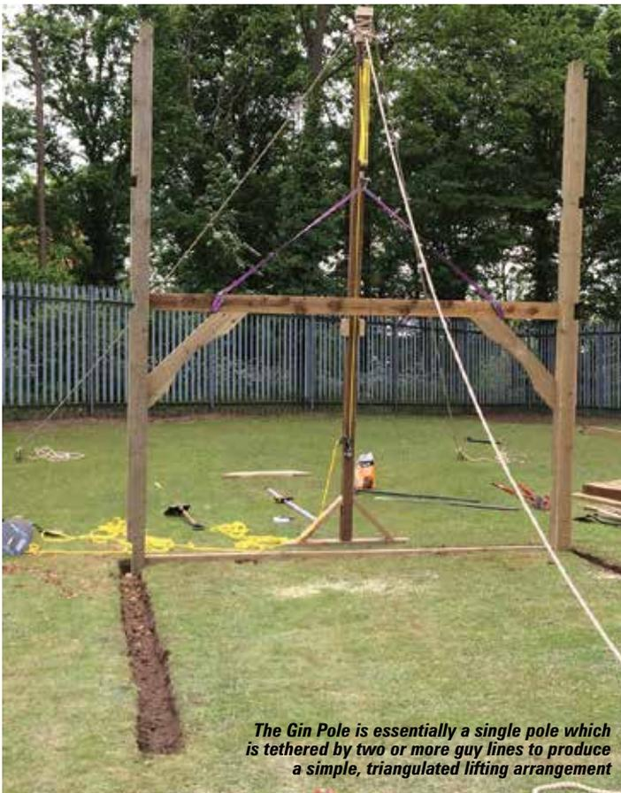
*The Gin Pole is essentially a single pole which is tethered by two or more guy lines to produce a simple, triangulated lifting arrangement*
