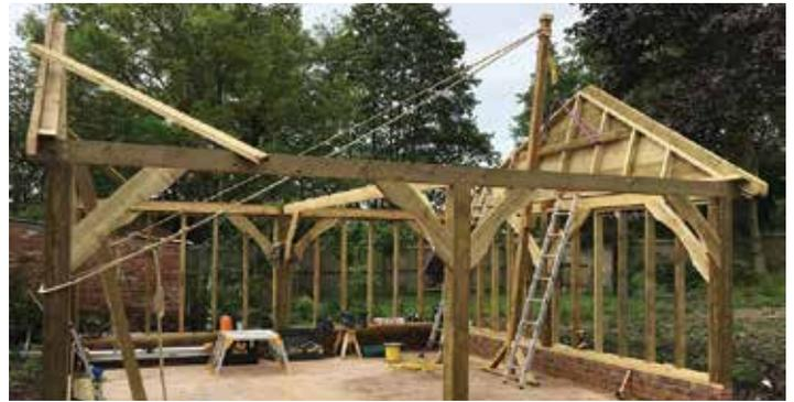
Frames weighing up to one tonne can be lifted.
