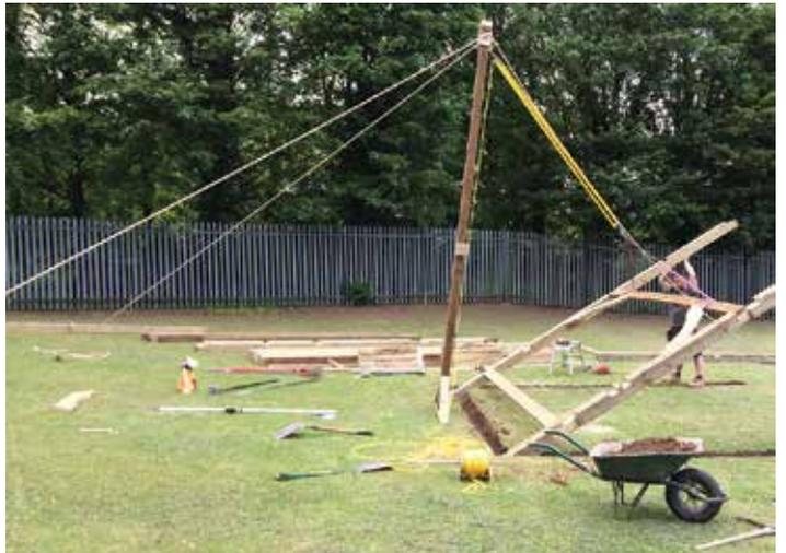
corresponding pole angle. Correctly rigged these adjustments may be undertaken while under load by the simple use of pulleys or hitches in the guy line system.
