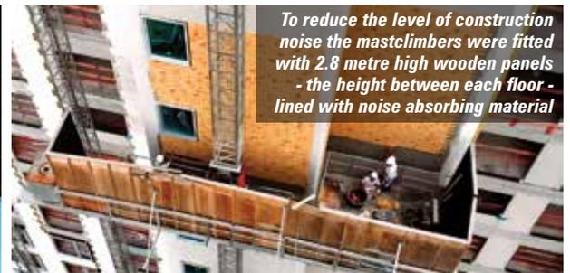
To reduce the level of construction noise the mastclimbers were fitted with 2.8 metre high wooden panels - the height between each floor - lined with noise absorbing material
