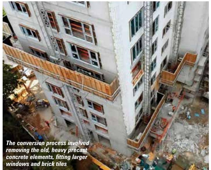
The conversion process involved removing the old, heavy precast concrete elements, fitting larger windows and brick tiles
