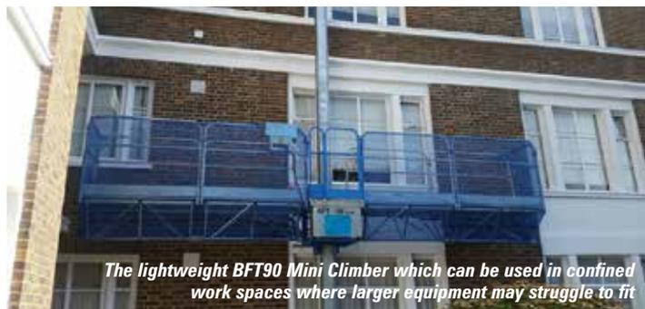
The lightweight BFT90 Mini Climber which can be used in confined work spaces where larger equipment may struggle to fit
