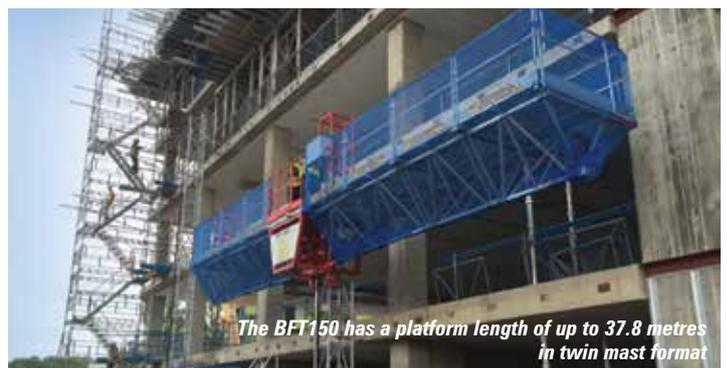
The BFT150 has a platform length of up to 37.8 metres in twin mast format
