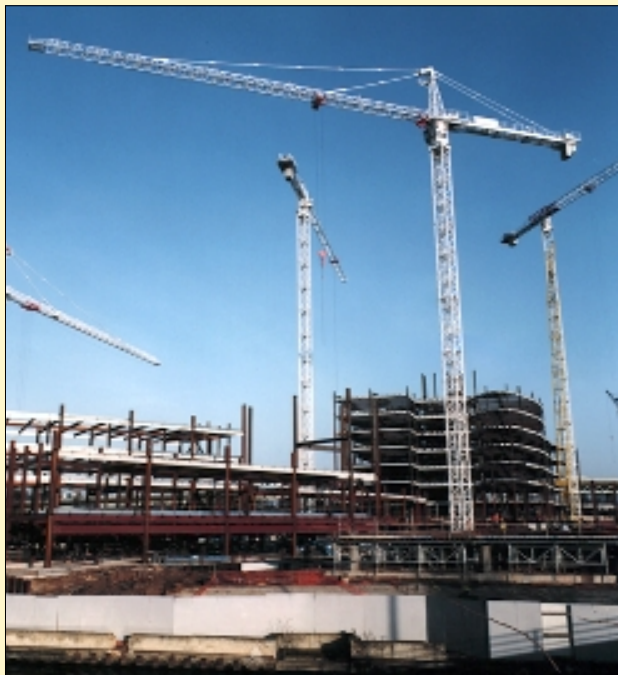
The new AC30 system from Cranesafe is designed to ensure that tower cranes do not collide. The electronic, networked system can monitor up to 20 luffing and saddle jib cranes on one site and is currently in use at Brentford.
