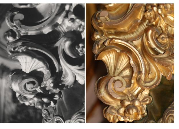
Figure 6. Audience room, east wall, gilded ornaments on the baldachin: losses and loosening of the gilded surfaces have not increased during the last 20 years
