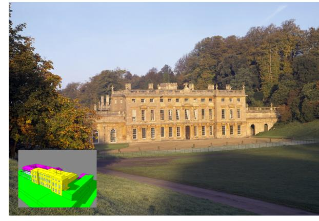
Solutions (IES) building simulation package. The remainder of the mansion was set to a background temperature of 16 °C. Test reference year climate data for the nearby town of Swindon were used as the weather input.
