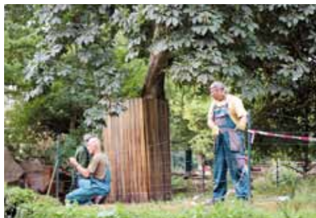
Likvidace škod po bouři dne 23. 6. 2017 Tiding away the damage after a storm on 23th June 2017
