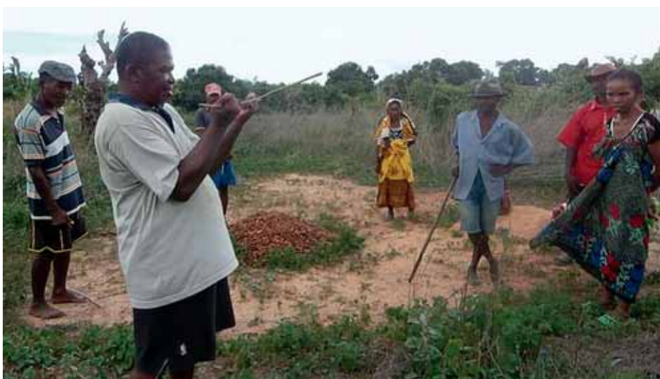
Stavba studny Digging out of a well
