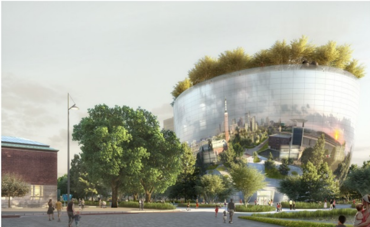
MVRDV's design resembles a sugar bowl, which means a narrow footprint can be combined with a generous terrace at the top. Image: Courtesy of MVRDV
