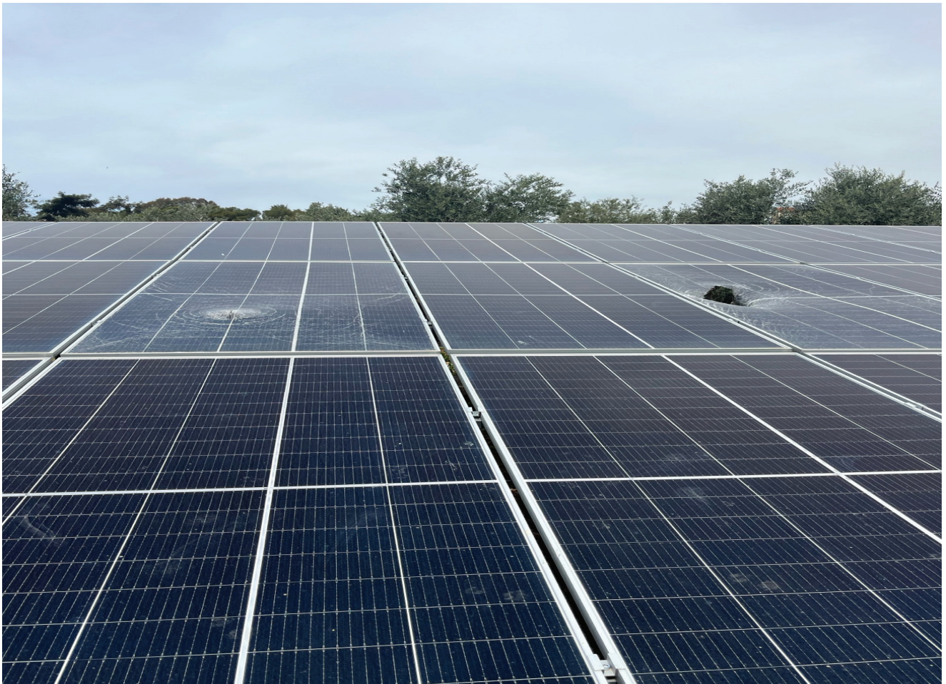
Figure 8. Damaged solar system in Nabatiyeh due to a nearby strike (source: author)
