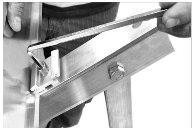
Tightening the upper clamps
