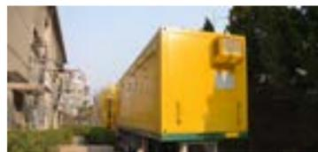
**40.5kV/12kV trailer substation**
