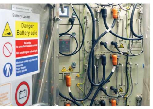
The battery room of the ferry- charging of the batteries takes place every time the ferry reaches one of the two ports.
