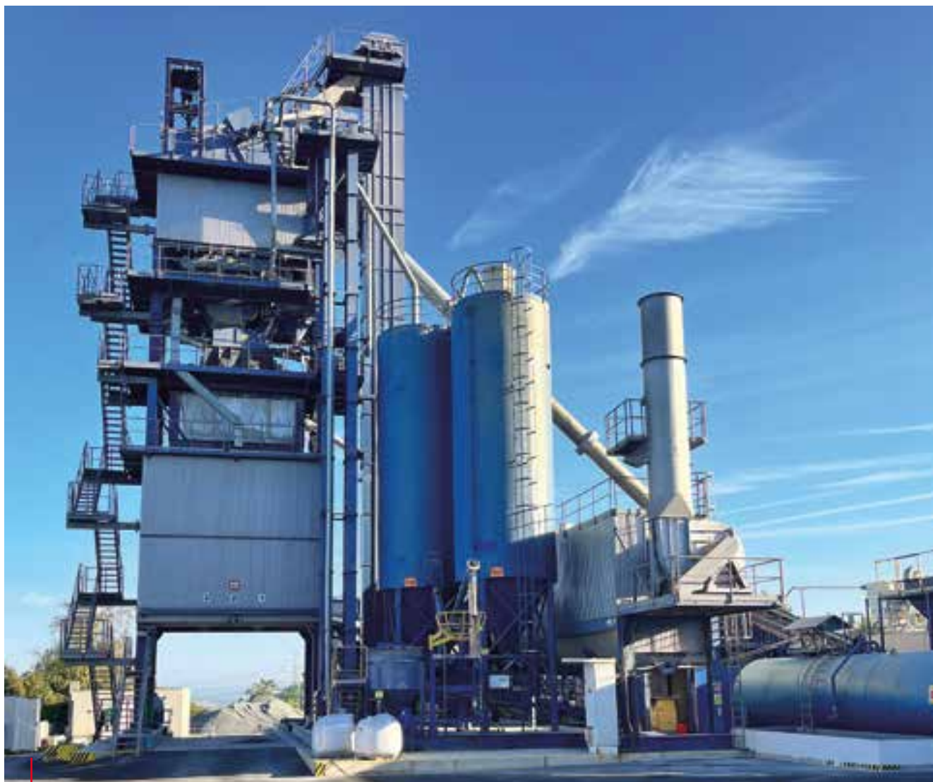
Obalovna Čenkov Čenkov Asphalt Mixing Plant
