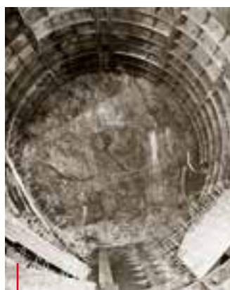
Stanice Můstek byla ražena metodou TBM, 1975 Můstek station was built using the TBM method in 1975
