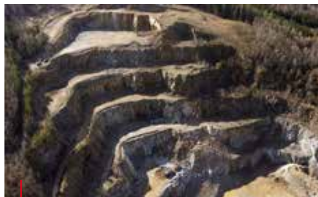
Kamenolom Mladovice Stone quarry Mladovice
