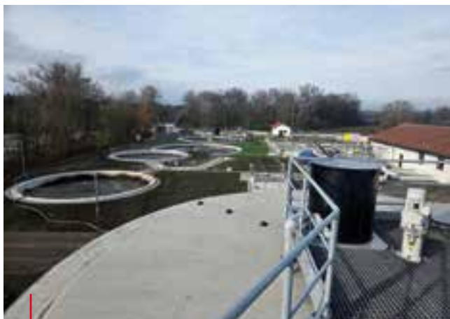
Rekonstrukce ČOV, Brandýs nad Labem Reconstruction of a wastewater treatment plant, Brandýs nad Labem
