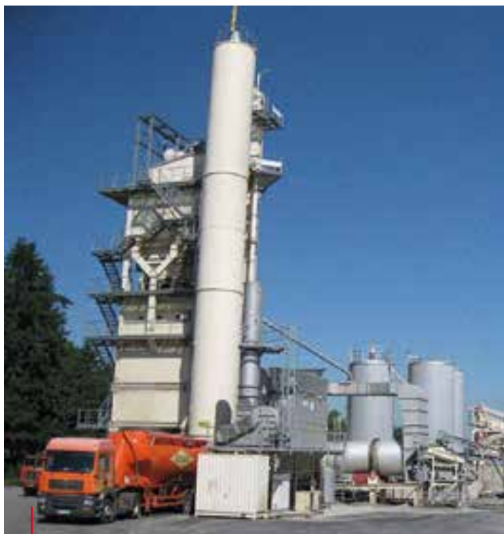
Obalovna Rančířov Rančířov Asphalt Mixing Plant
