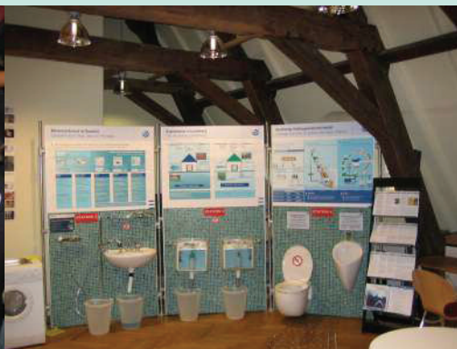
Experimental installation “Wasserwerkstatt” realised in collaboration with the Service National de la Jeunesse (SNJ, Centre Hollenfels) and financed by the FNR
