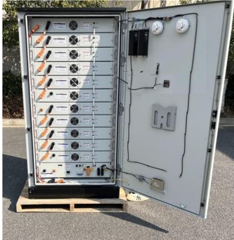
Pic 5 Internal view of Viessmann Battery Solution CS112
