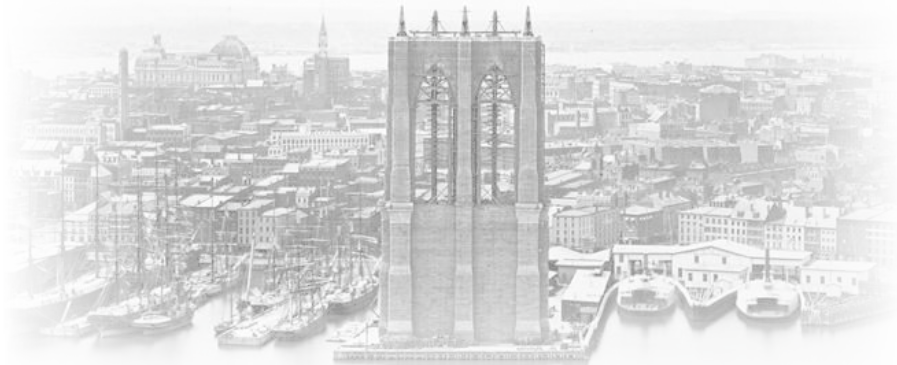
Building the Brooklyn Bridge
