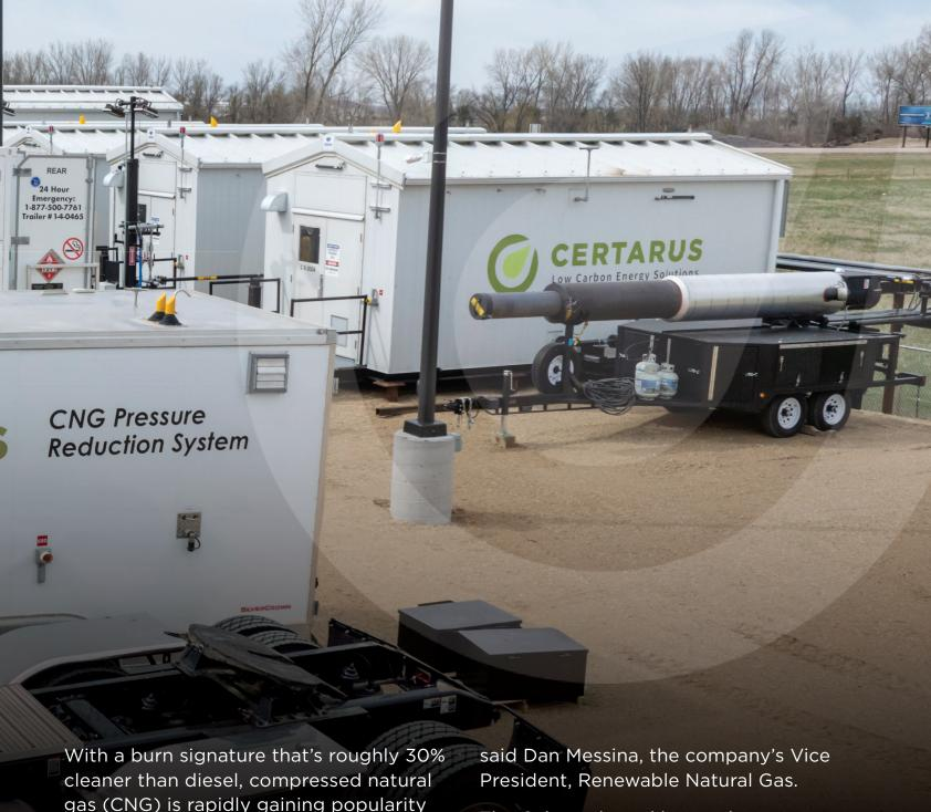
gas (CNG) is rapidly gaining popularity as a replacement fuel for a plethora of industries. Natural gas innovator Certarus was a catalyst for the oil and gas sector to move away from running diesel for the onsite energy demands of drilling and completions operations.
