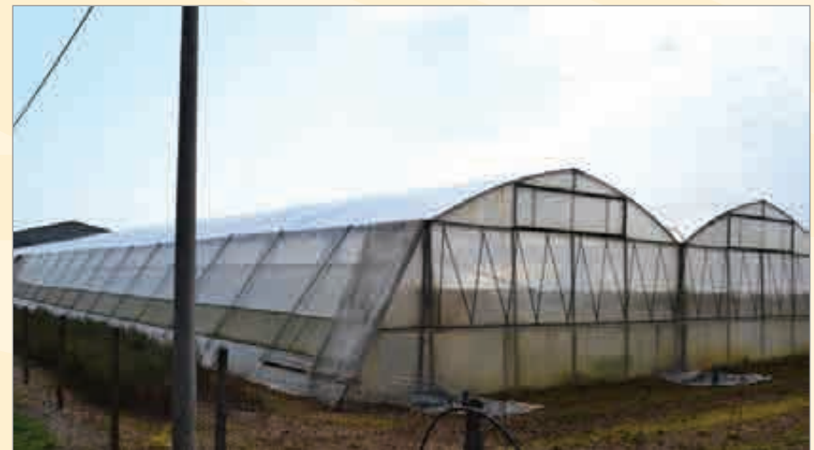
Plastenici Green houses
