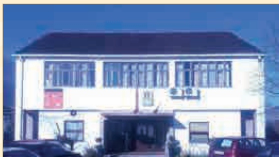
Upravna zgrada Administration building
