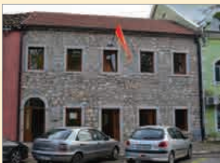
Upravna zgrada Administration building
