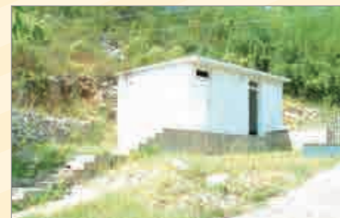
Pumpna stanica Pumping station
