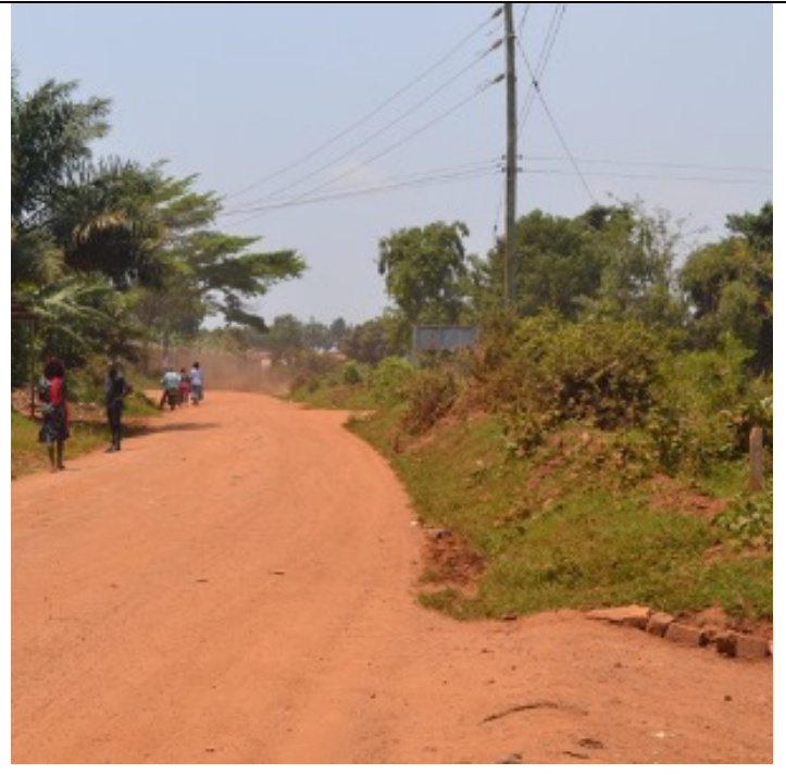
Plate 4: Access road that requires to be widened for safe vehicle passage
