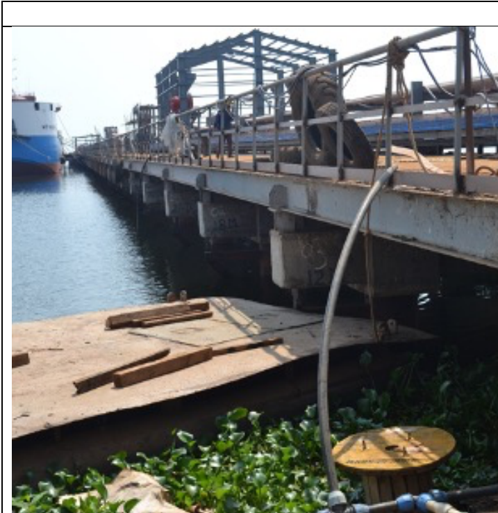
Plate 1: Jetty (under construction)
