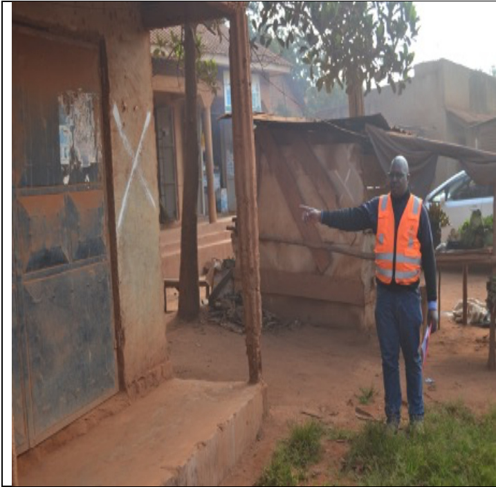
Plate 5: House adjacent to the road that will need to be moved for road widening
